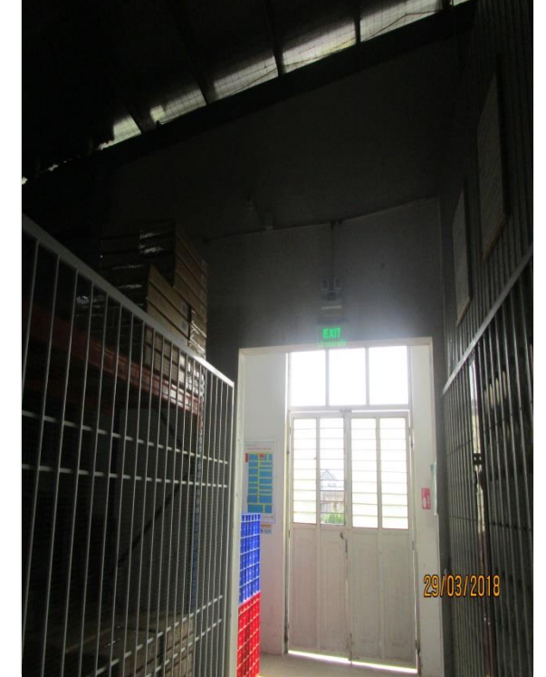
Secure door to building
